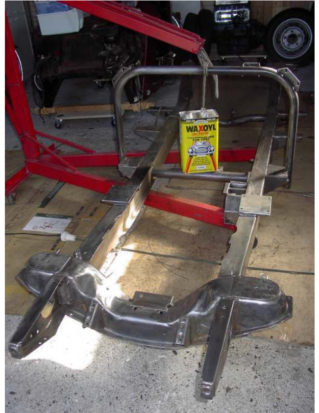
Using Waxoyl to protect the box section.
