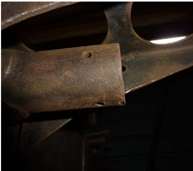
PHOTO 1 – Near side showing original and later pin positions.
